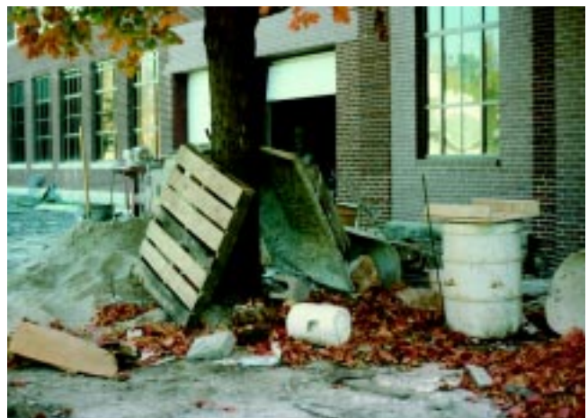
Soil compaction and direct injury to tree from construction activities.
